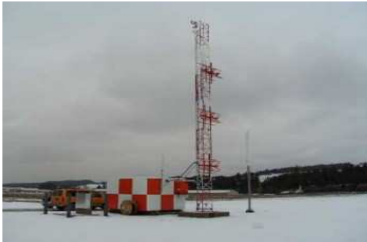
Figure 10: ILS-GS antenna
