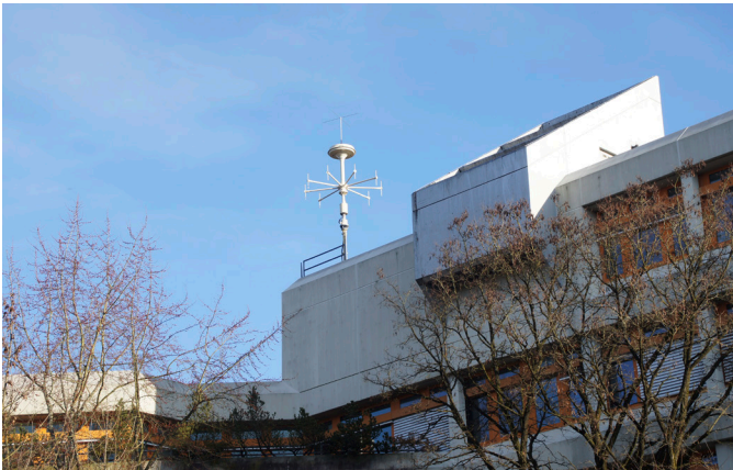
One of the BNetzA's direction finding stations installed in Grünwald near Munich, Germany.
