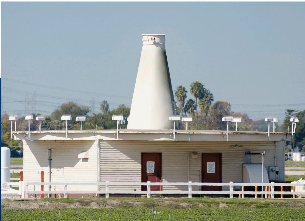
A state-of-the-art TACAN beacon tower.
